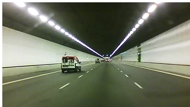
Fig. 2. Typical tunnel expressway in Singapore.
