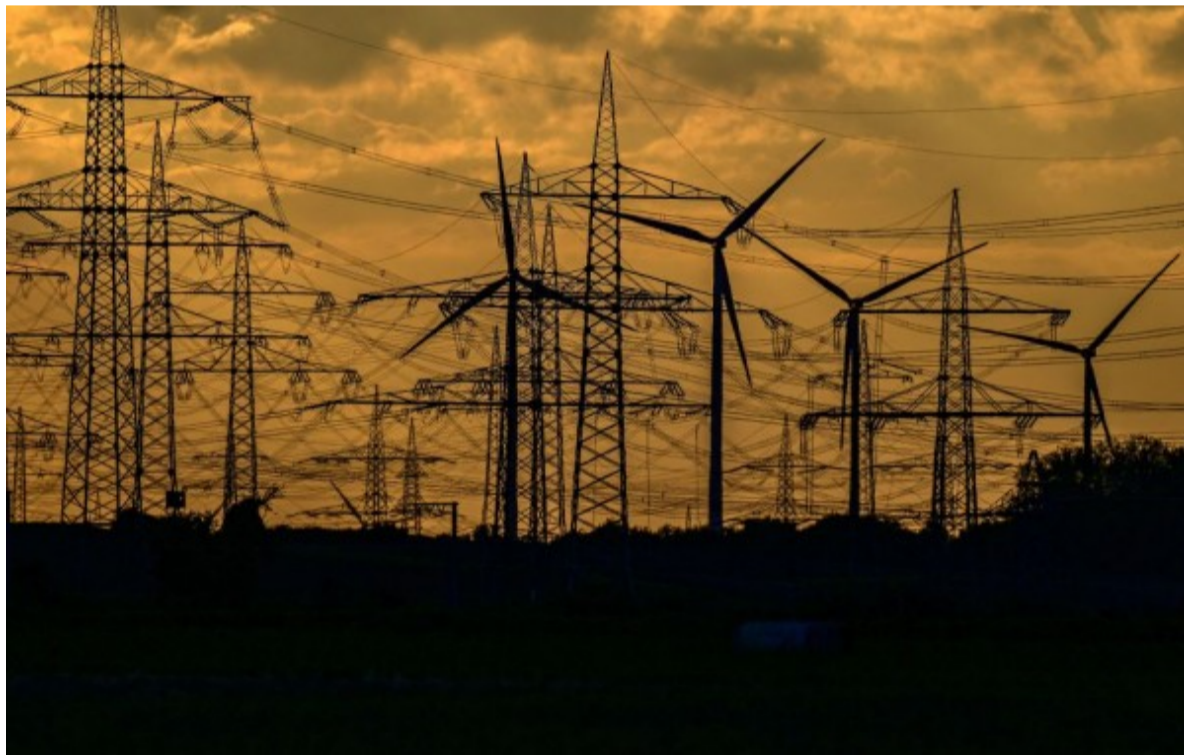
(Photo : INA FASSBENDER/AFP via Getty Images) This picture taken on October 5, 2022 shows wind turbines and power pylons near Neurath, western Germany. - German energy provider RWE brought forward its exit from coal power to 2030 on October 4, 2022 amid fears the country's plans to abandon fossil fuels are wobbling following the energy crisis caused by Russia's war in Ukraine.
