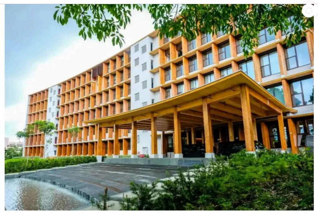
Mold appeared in the "Earth Chamber" more than a year after it was put into use. After experts evaluated the building, they believed that condensation and rain were the main causes of the mold problem in the building, and had nothing to do with the main material of the building, wood.
