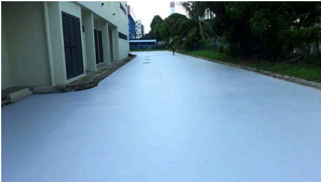
Image: The road pavement of the test-site in Singapore with cool paint coatings. Credit: NTU Singapore
