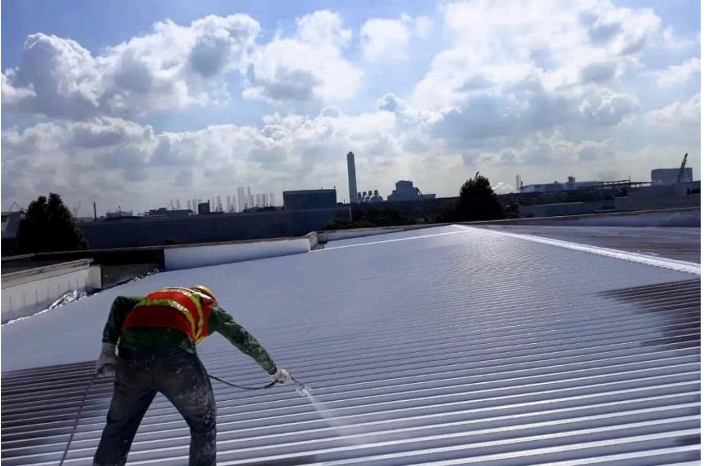
The NTU team coated the roofs, walls and a road of an industrial area with cool paint for the trial. PHOTO: NTU
