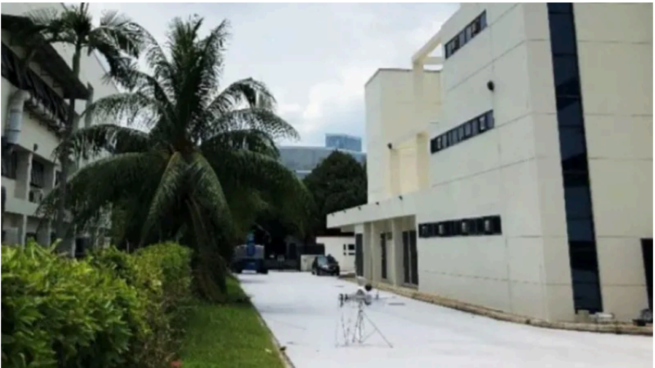
The road, pavement and walls of the test-site in Singapore with cool paint coatings - NTU Singapore
