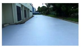
Image: The road pavement of the test-site in Singapore with cool paint coatings.
