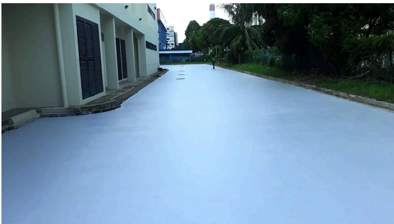
The road pavement of the test site in Singapore with cool paint coatings. Nanyang Technological University
