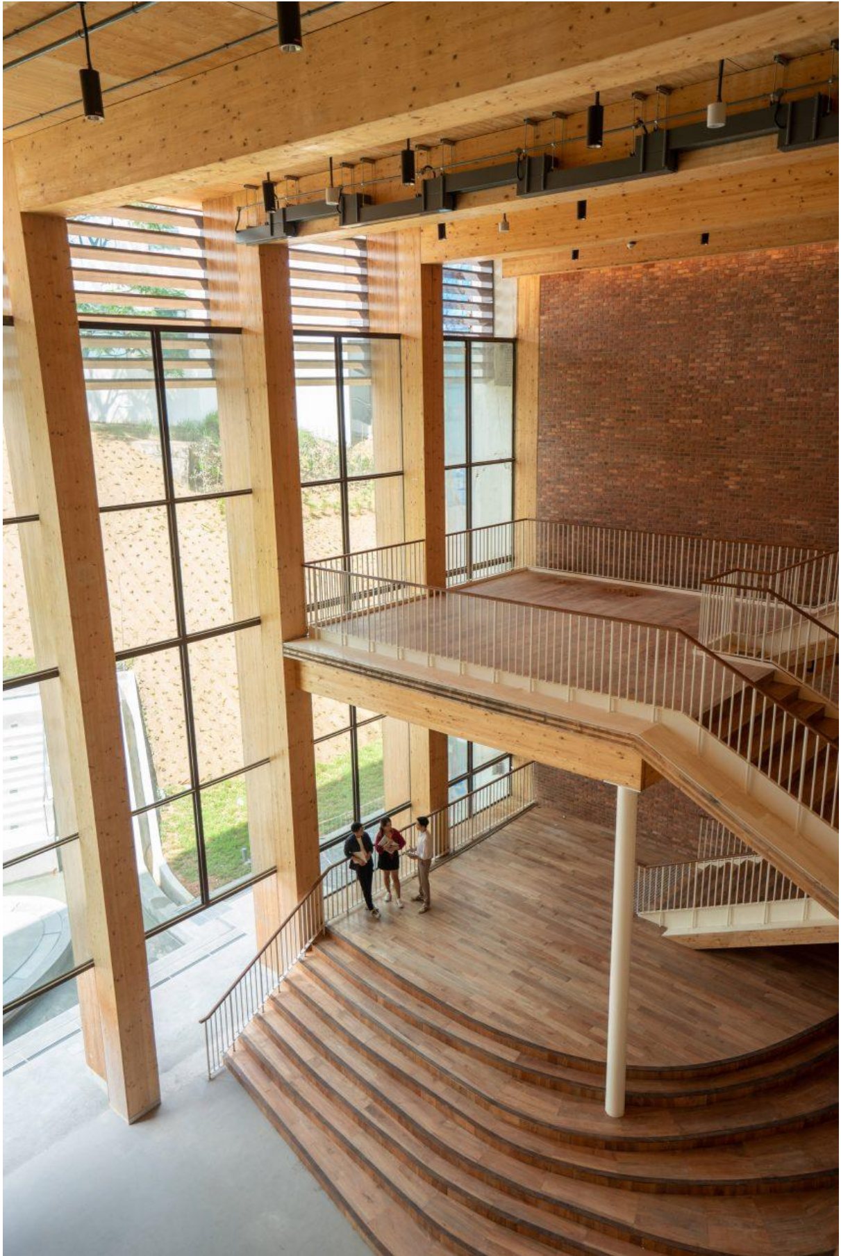
Its timber structure is exposed throughout
