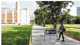
A footpath at Our Tampines Hub constructed from Newsand, which is made from repurposed solid waste, and is a crystal-like substance resembling sand. Reducing the amount of sludge produced and recovering more usable resources from it is another area Newri is looking at. ST PHOTO: ONG WEE JIN
