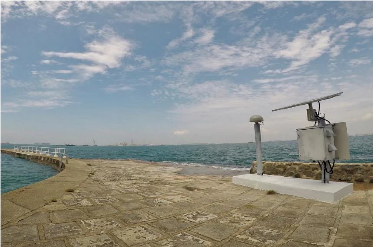
One of the SLA's nine Singapore Satellite Positioning Reference Network stations. PHOTO: SINGAPORE LAND AUTHORITY
