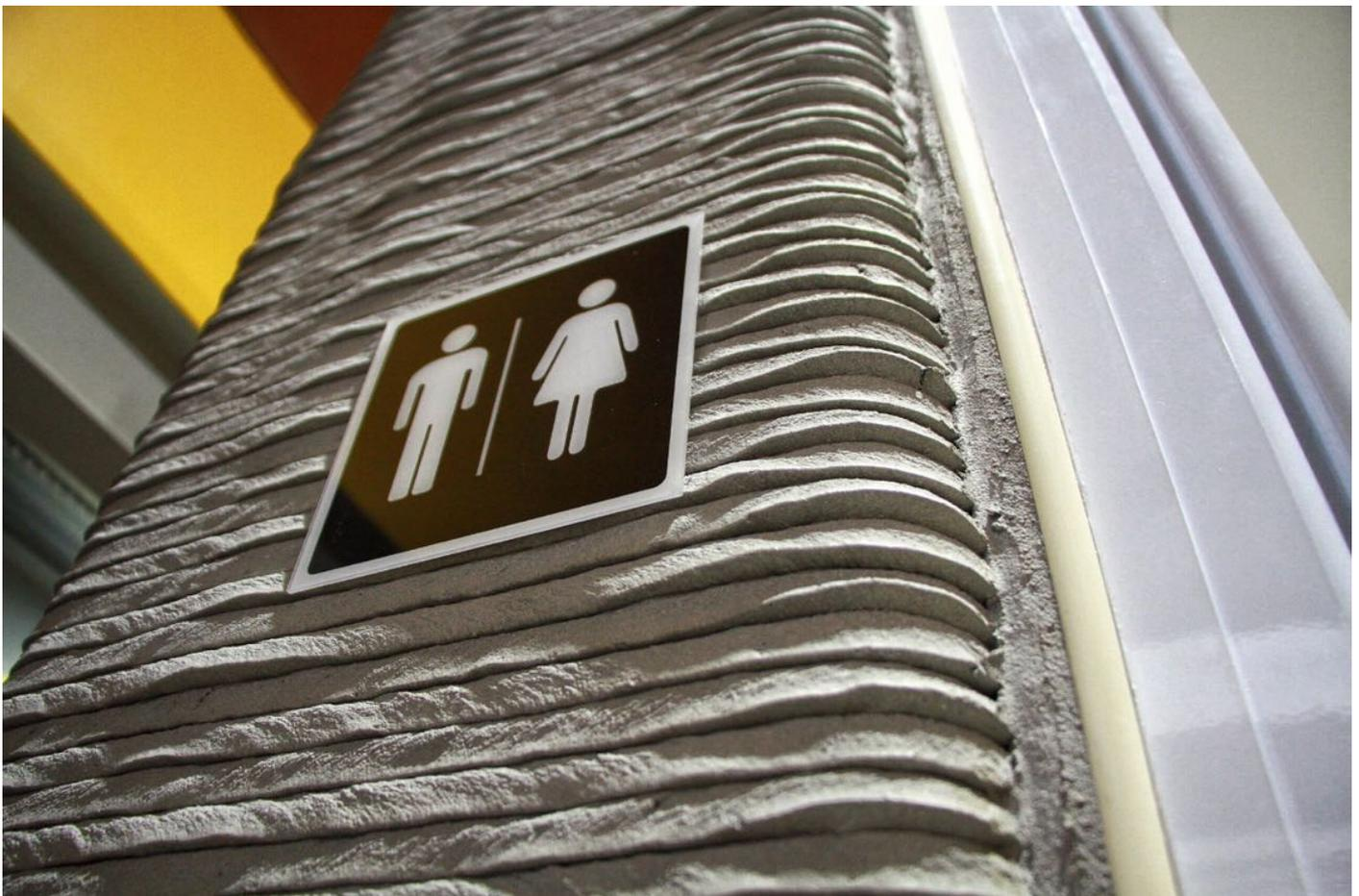
*A closer look at the prefabricated bathroom unit's texture, which was formed by repeated layers of the W-lattice shape. Photo: Neo Rong Wei/TODAY*
