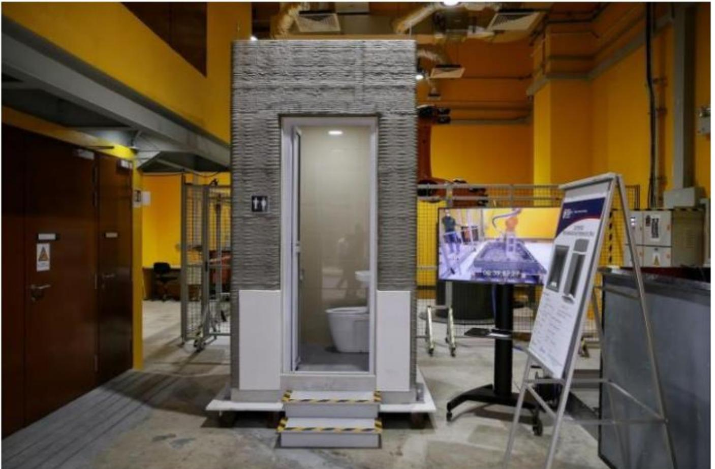
The technology could potentially help firms build prefabricated bathroom units that are 30 per cent lighter than current models using one-third less time. ST PHOTO: KEVIN LIM
