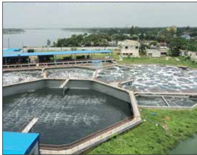
Flagship EcoSystems' Dhaka EPZ central effluent treatment plant is the largest of its kind in Bangladesh. PHOTO: FLAGSHIP ECOSYSTEMS
