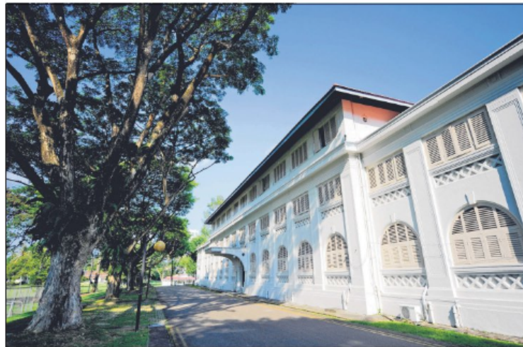
This conservation building next to Tan Tock Seng Hospital will be the base for Singapore's third medical school. The school, jointly managed by Nanyang Technological University and London's Imperial College, is expected to open in 2013. ST PHOTO: BRYAN VAN DER BEEK
