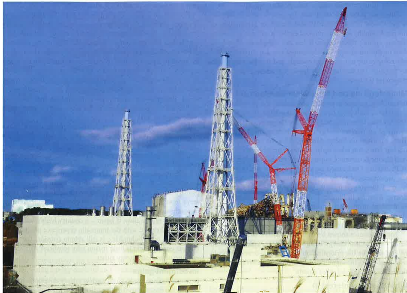
A general view of the Fukushima Daiichi site taken in December 2012. The light blue building in the centre is Unit 2. Behind it is Unit 1, which has been covered by a new structure with a peaked roof. The tangled mass of metal and rubble is Unit 3. The top of Unit 4, whose damaged upper levels have been removed, is visible towards the right of the picture. In the distance, to the far left, stand the undamaged Units 5 and 6, which were built on higher ground and escaped the worst of the tsunami.
