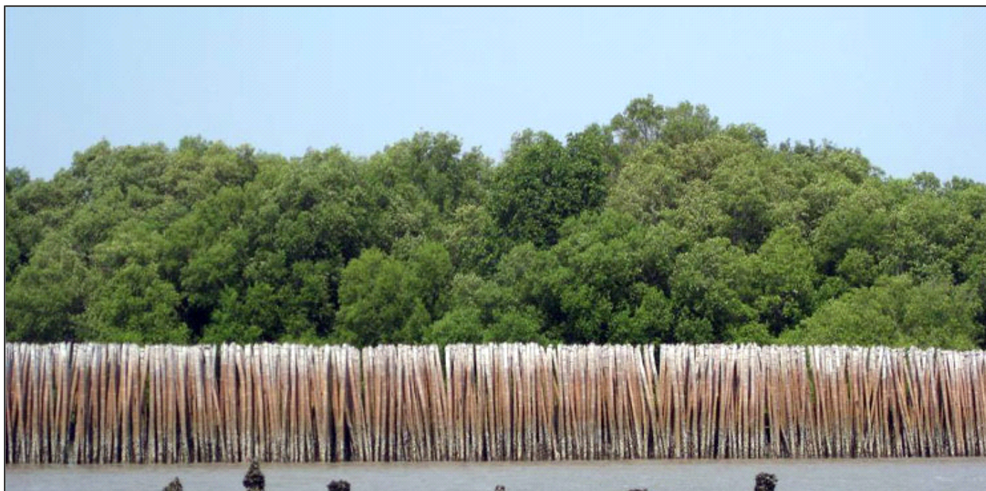
A bamboo dike built by residents in Bang Khun Tian to prevent coastal erosion and sustain their aquaculture livelihoods.
