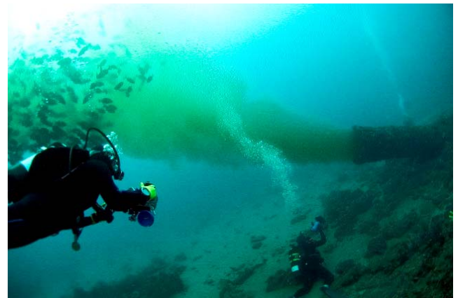
Submerged marine outfall
