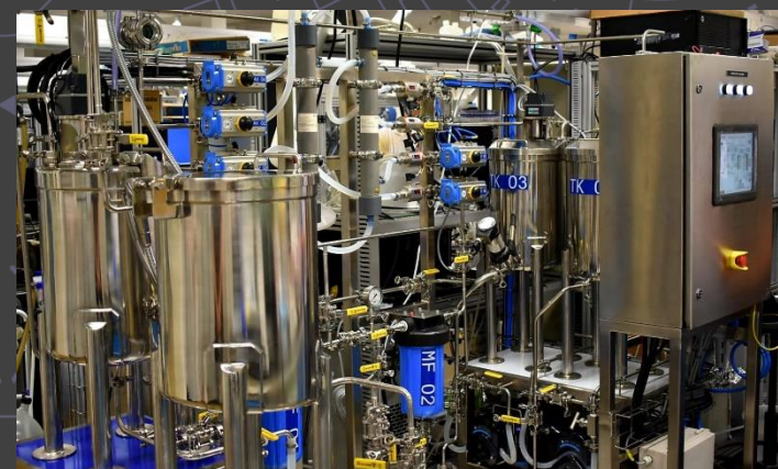
The pilot system utilising the membrane technology in the forward osmosis (FO) process, developed in NEWRI laboratories.
