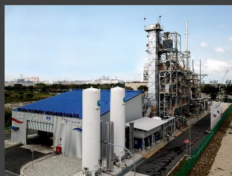
Waste-to-Energy Research Facility (WTERF)
