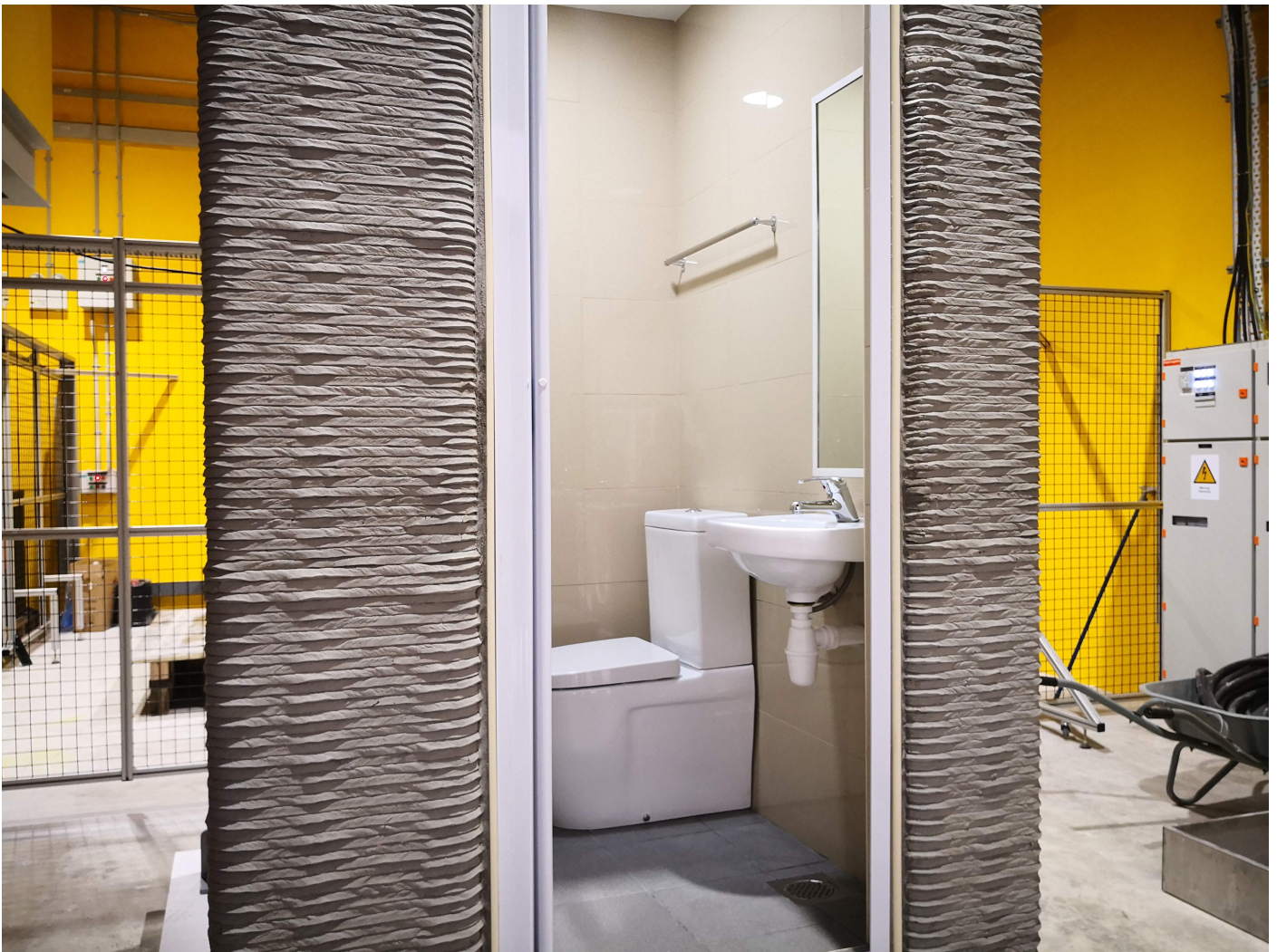
The 3D-printed bathroom unit could be fitted with all the necessities of a typical toilet, including ceramic tiles and flooring. NTU Singapore
