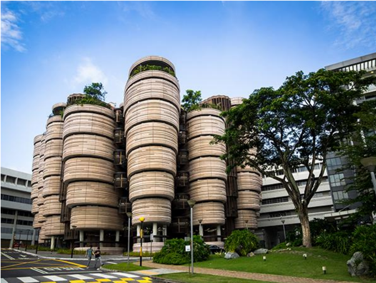
The Hive, also known as the Learning Hub, is a building located in Nanyang Technological University
