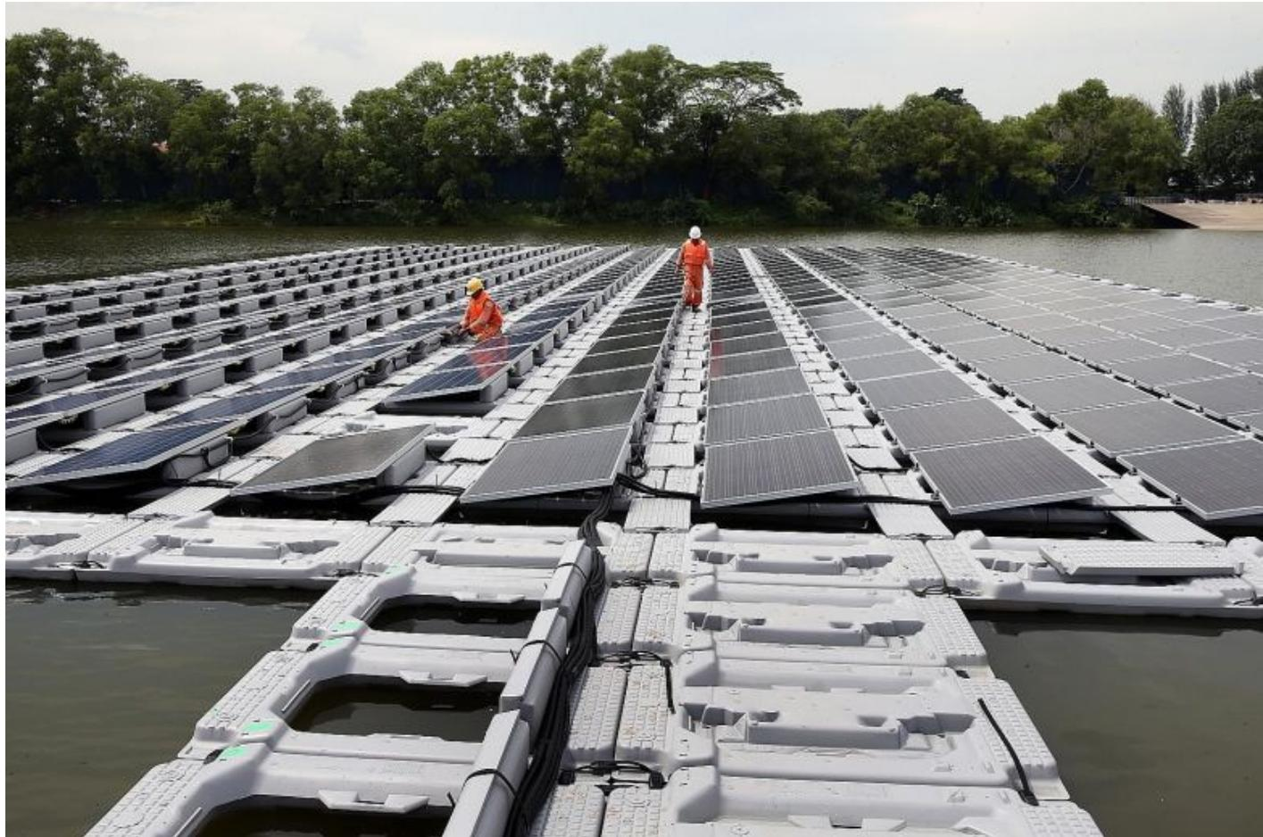
The floating solar panel test bed at Tengeh Reservoir was launched last year to study different photovoltaic systems. Solar energy is important to Singapore since other forms of renewable energy are not as viable here. ST FILE PHOTO
