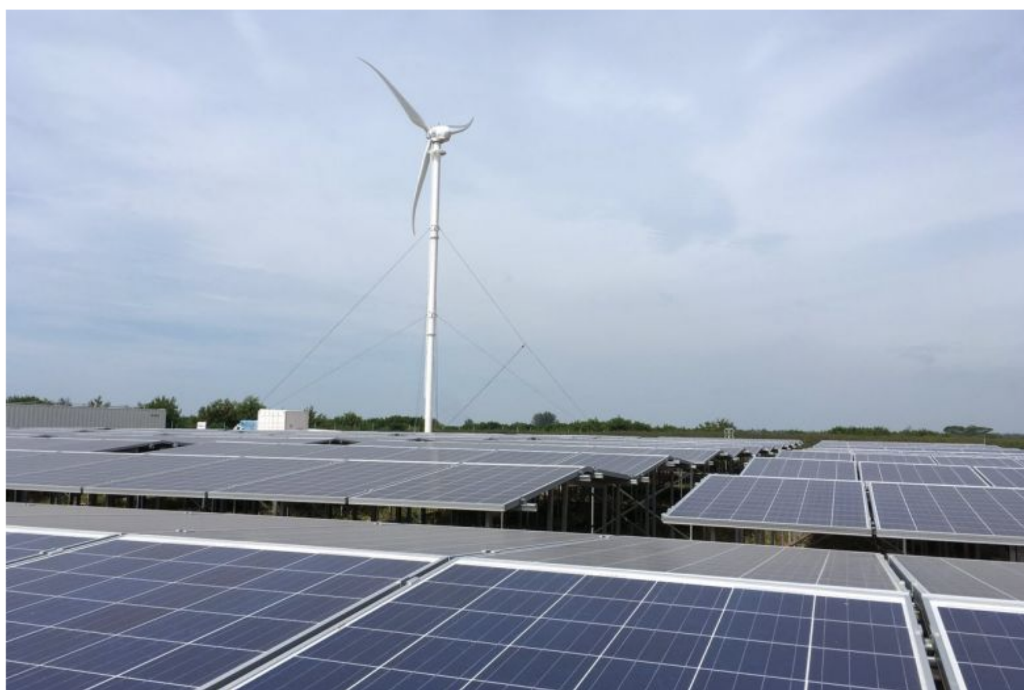
The turbine is one of up to seven which will generate power for hybrid microgrids on the landfill south of Singapore, together with other sources such as photovoltaic (solar) panels. ST PHOTO: ALPHONSUS CHERN
