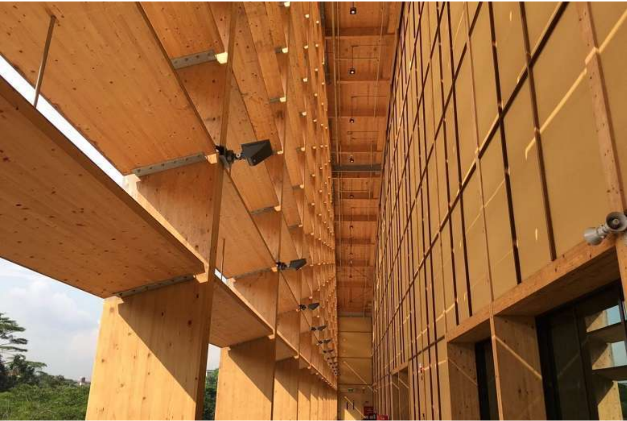
The new NTU sports hall, called The Wave, is the first large-scale building in South-east Asia with a structure built completely using mass-engineered timber. ST PHOTO: ONG WEE JIN
