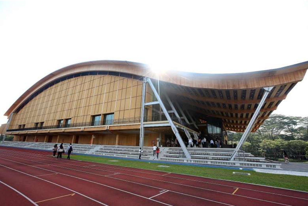
The Wave, NTU's new sports hall, is made mostly of mass engineered timber. The prefabrication of parts led to speedier construction and yielded a 25 per cent savings in labour. ST PHOTO: ONG WEE JIN
