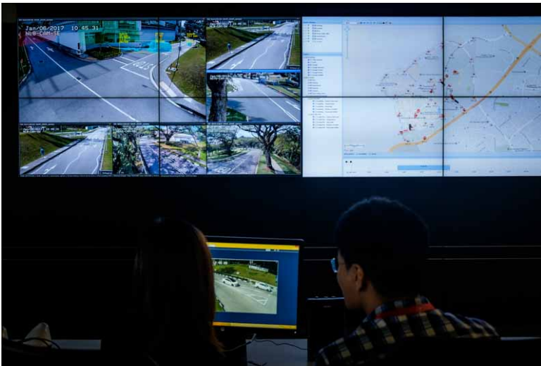
Above photo: Control centre of NTU-NXP Smart Mobility Test Bed. Photo credit: NTU
