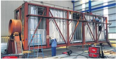
**1.** Each time, 40-50 empty modules manufactured in prefabrication plants in China are shipped to Singapore. They have floor tiles, windows, internal door frames and internal boards installed.
