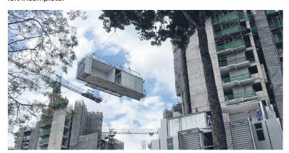
**3.** Every day, about 6-8 modules are delivered to the construction site to be lifted and assembled. Only after they are hoisted up are the sanitary drainage pipes connected manually to the units below them until everything is linked to the main drainage vertical stack. Mechanical and electrical services and floor tiling are then installed along the corridors to complete the project.
