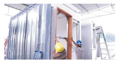
2. Modules arrive in Singapore's ports and are transferred to fit-out yards. Modules have to be fitted out within 1-2 weeks with lights, electrical wiring, sprinkler pipes, switches, fans, toilet piping, hot water supply, toilet floor casting and tiling, doors etc. Only the water closets and basins are left incomplete.
