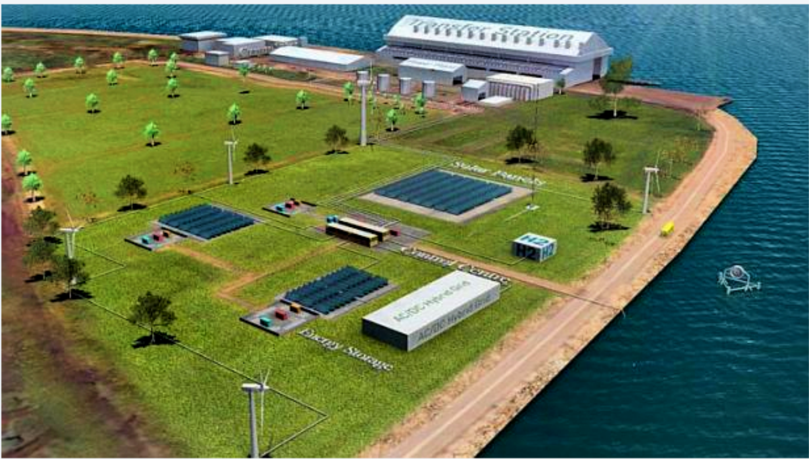
An artist's impression of the hybrid micro-grid that will be built offshore at the Semakau Landfill. -- PHOTO: NTU
